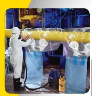
It safely encloses pipe diameters from 10" to 14".
